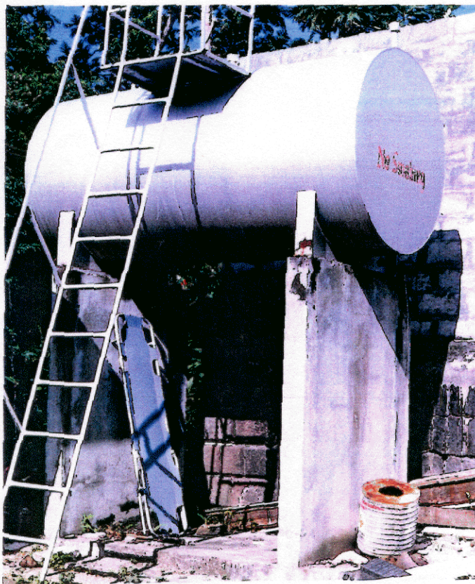
PHOTO 49 GASOIL STORAGE TANK AT CREMATION PLANT
