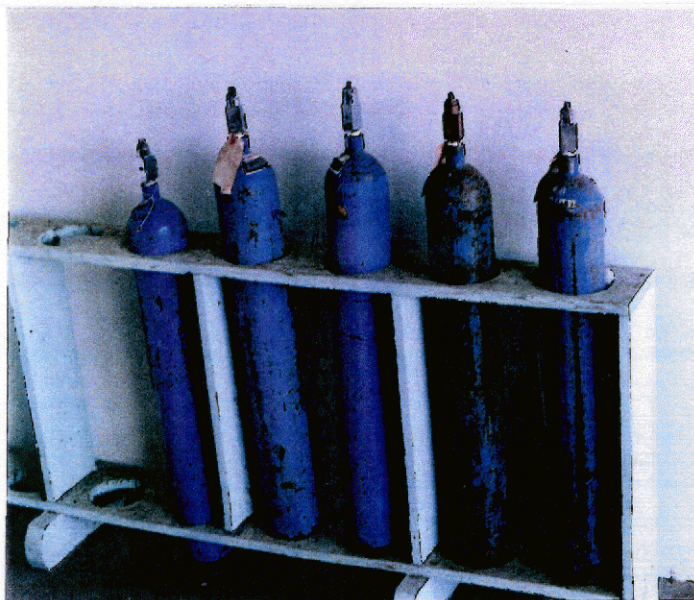
PHOTO 52 ADEQUATE DISPOSITION OF GAS CYLINDERS
