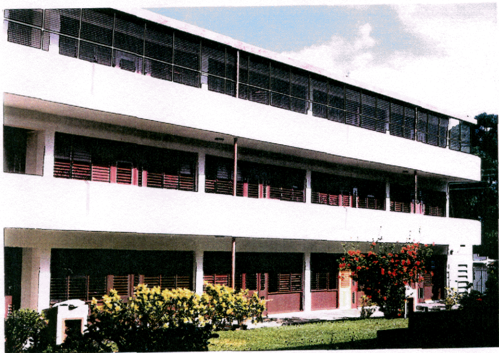
PHOTO 18 WESTERN FACADE OF BUILDING H. THE RED VERTICAL PIPES ARE RAIN WATER DRAINAGE (SEE DETAIL IN PHOTO 19)
