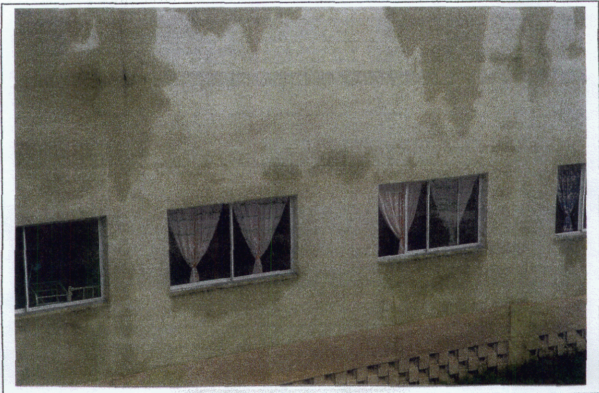
Photo 20 - External wall of the Hospital Note the retained damp and the cracks around the perimeters of wall panels.
