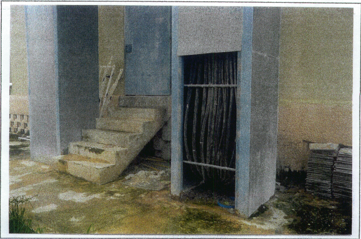
Photo 23 - Electrical Cable Duct
