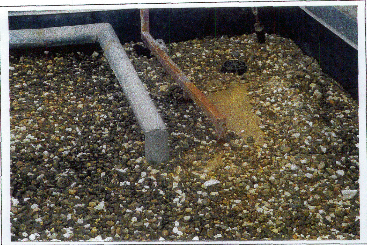
Photo 27 - The roof of the Utilities Block Water collects under the waterproofing membrane.
