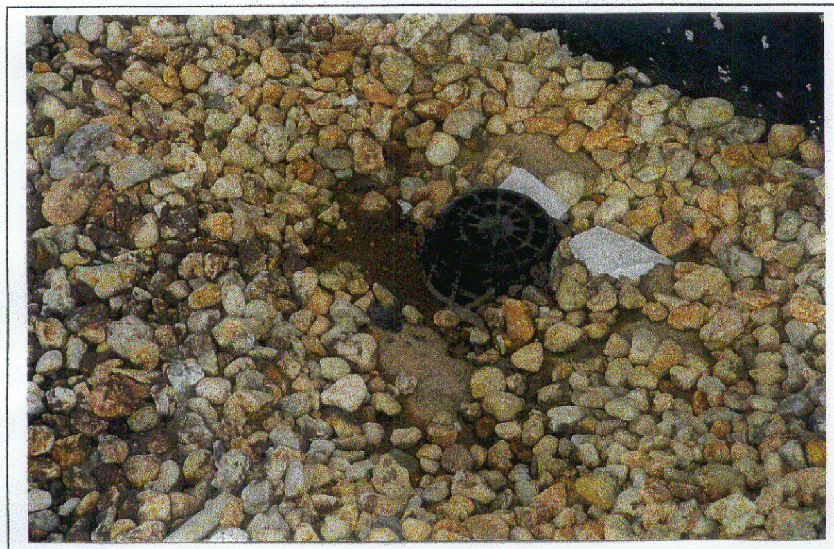
Photo 6 - Drain inlet on the roof of the Hospital Some leaks are traced to these locations
