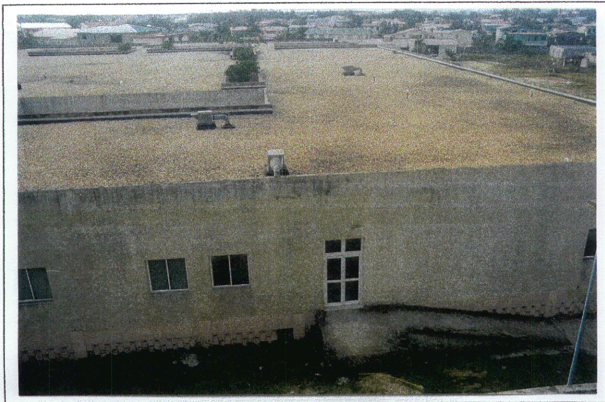
Photo 5 - The roof of the Hospital covered with gravel ballast The gravel poses a hazard to windows in high winds It is intended to remove the gravel as part of the EU Rehab project
