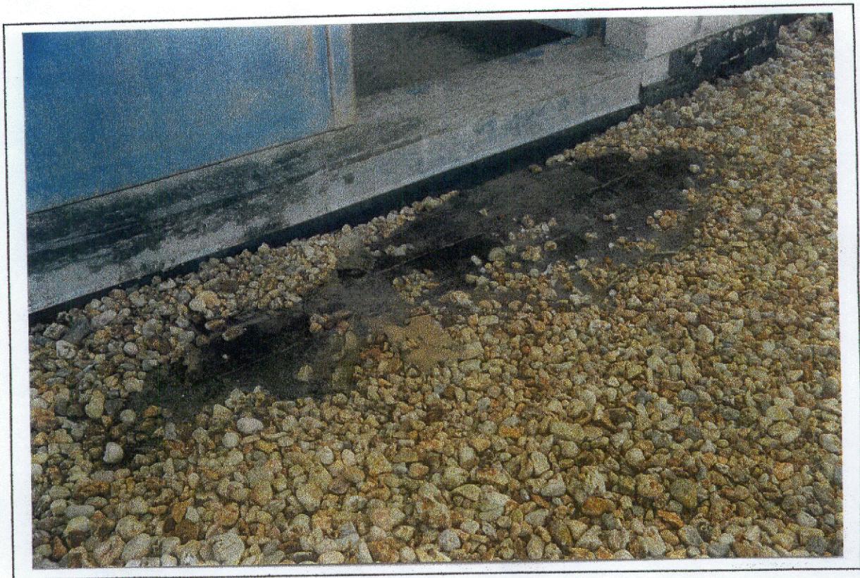
Photo 7 - Edge flashing on the roof of the Hospital Some leaks are traced to these locations
