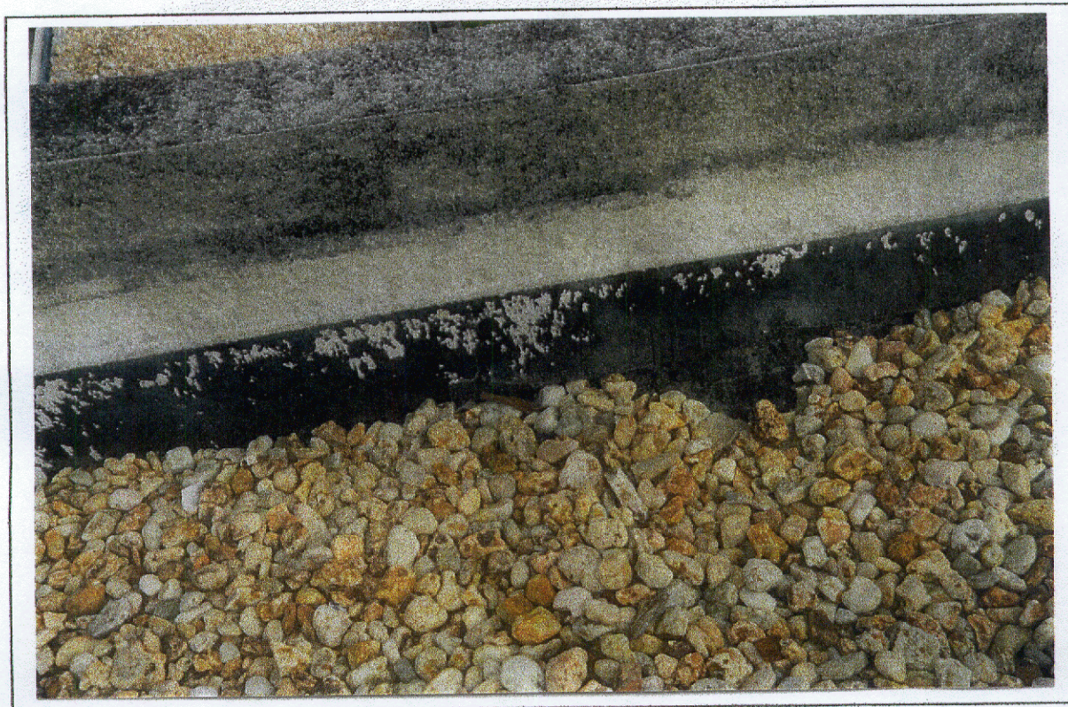
Photo 8 - Edge flashing on the roof of the Hospital Some leaks are traced to these locations
