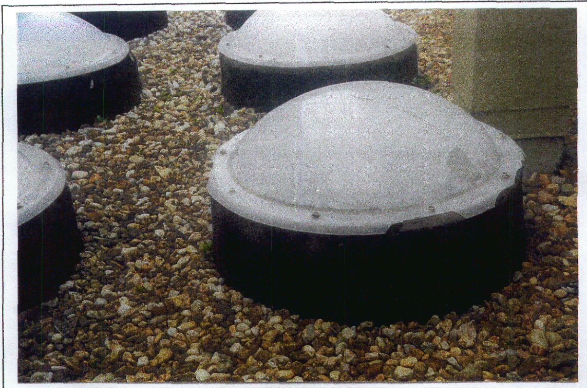
Photo 9 - Cracked skylight
