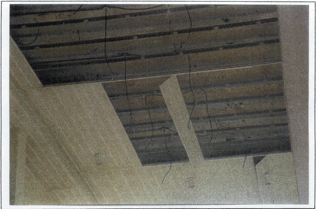
Photo 11 - Suspended ceiling at the entrance to the Hospital A large proportion was removed during the passage of Keith
