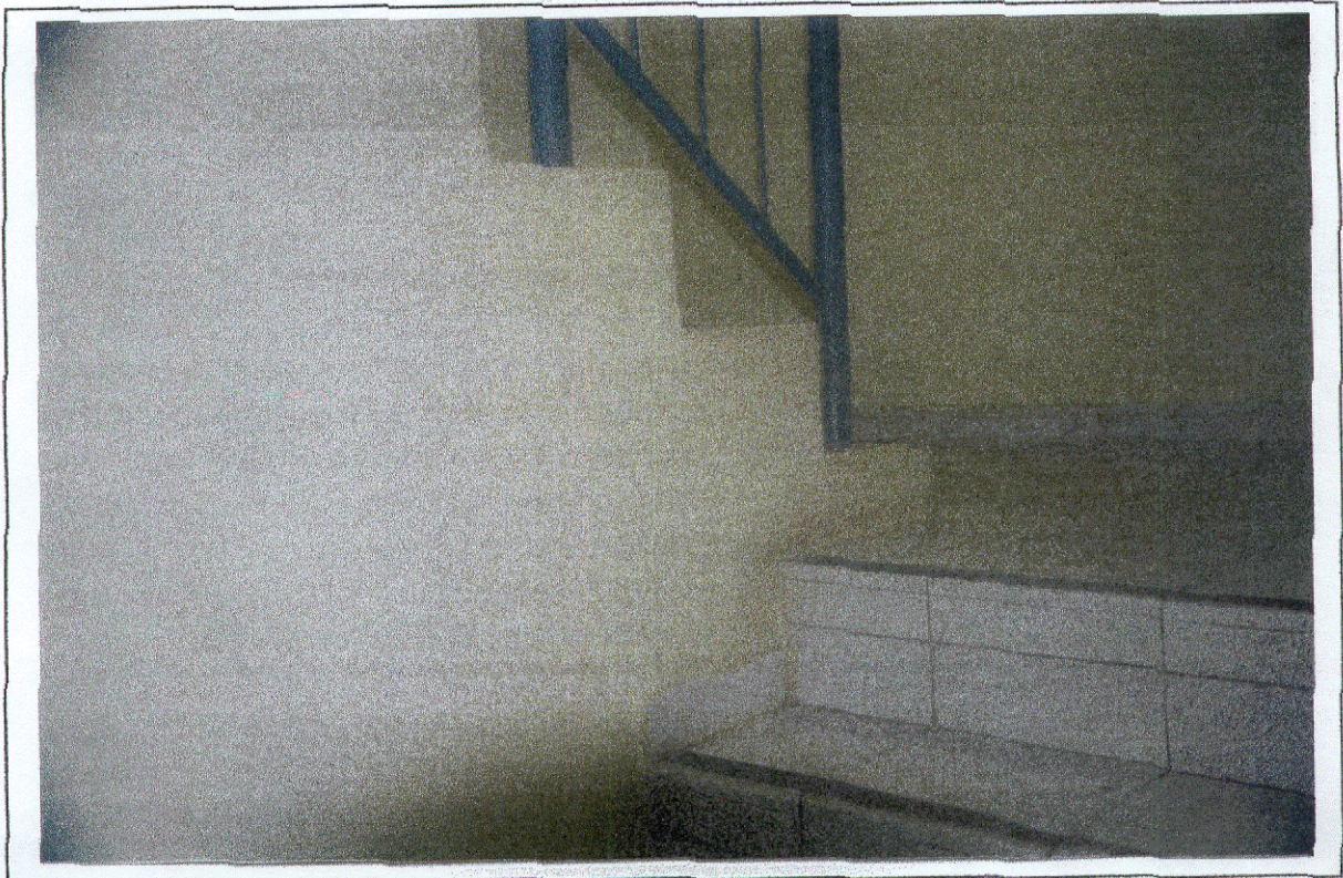
Photo 18 - Staircase in the Hospital Note the irregularities in the heights of adjacent steps. This is dangerous, especially in a hospital.
