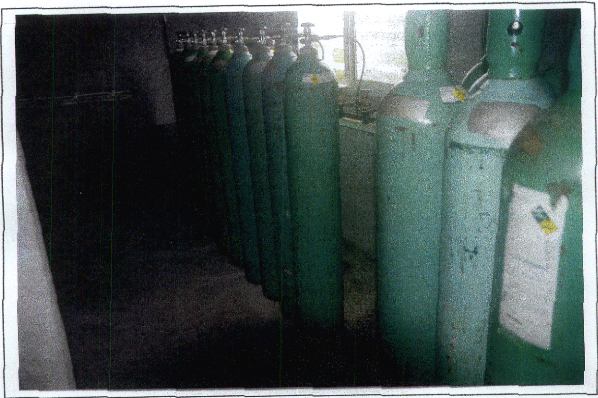
Photo 17 - Medical gases in unsecured cylinders These require restraints to prevent them from toppling in earthquakes.
