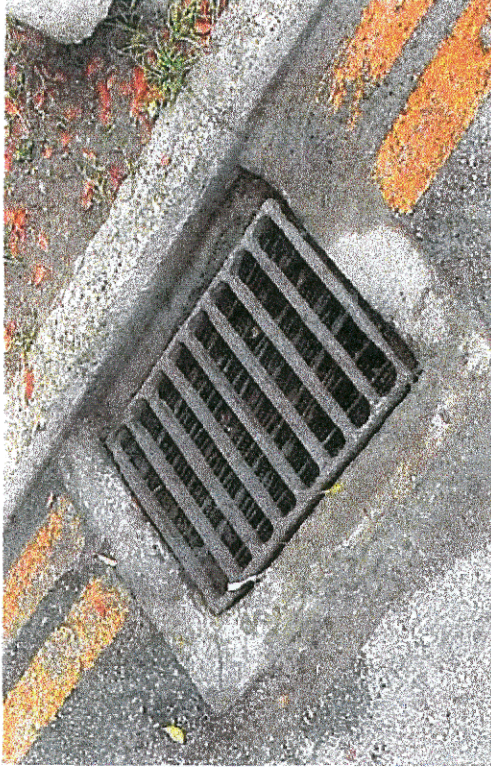
Photo 41. One-way avenue to the East of the site. A drainage grille combined with a fine mesh to collect debris is used for stormwater drainage.
