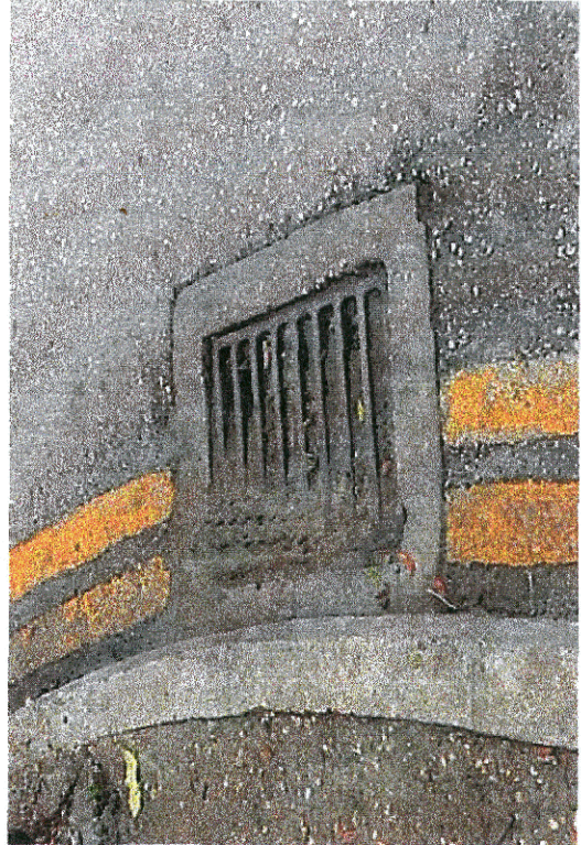
Photo 41. One-way avenue to the East of the site. A drainage grille combined with a fine mesh to collect debris is used for stormwater drainage.
