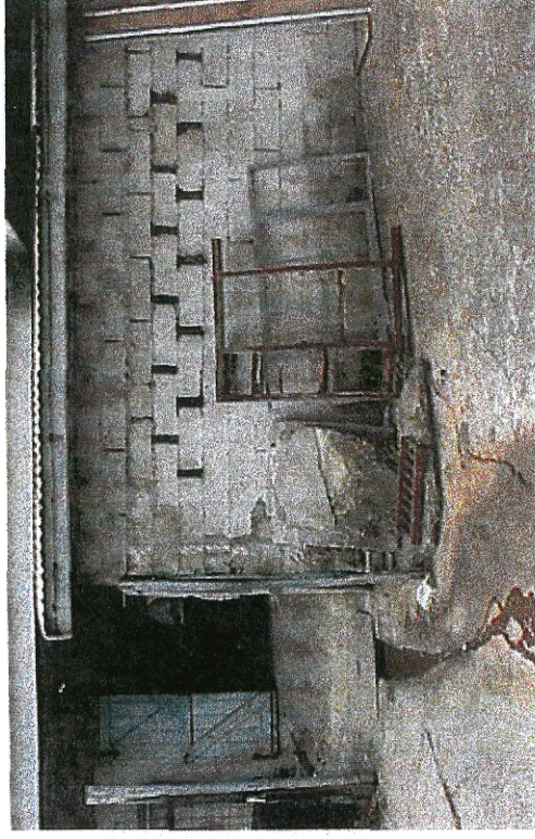
Photo 7. Small shed on the North end of Workshop #1. The workmanship of the horizontal courses of the mortar joints between blocks is poor.
