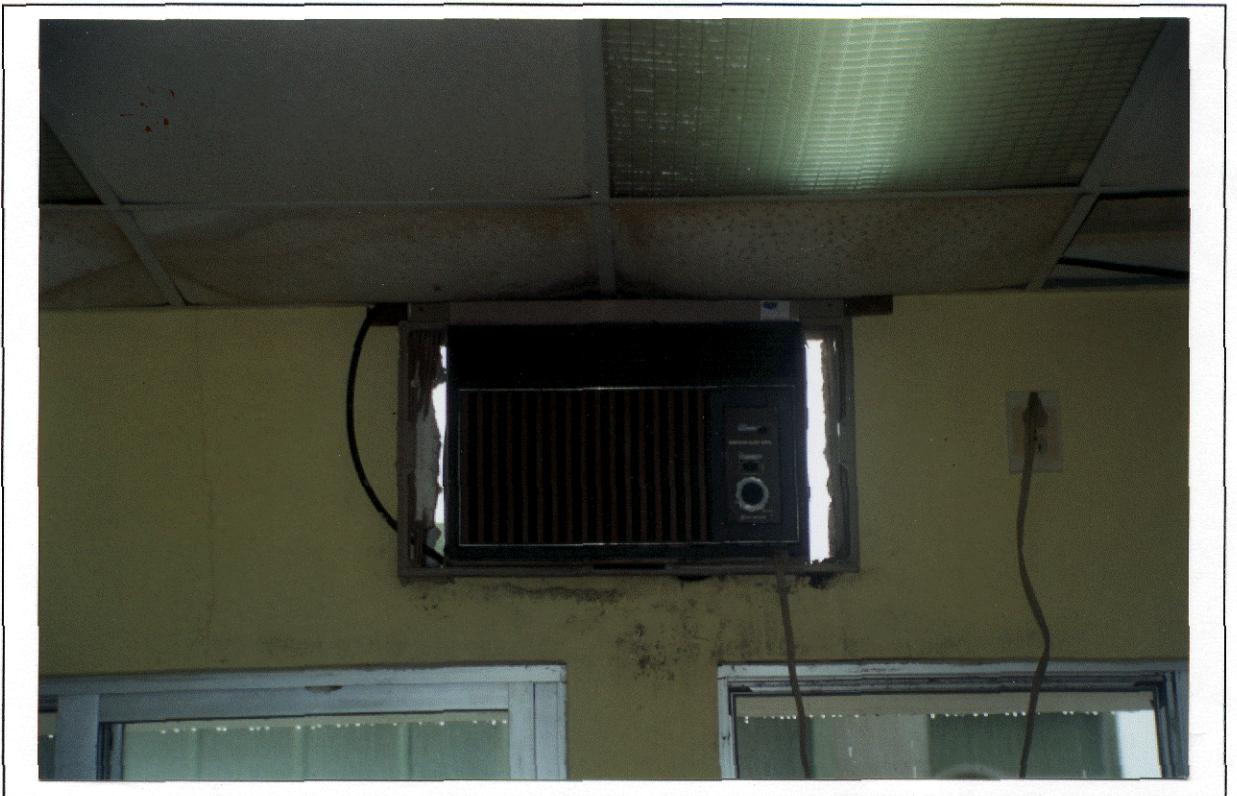
Photo 20 - Histology Large gaps between AC unit and wall allows significant ingress of rain.
