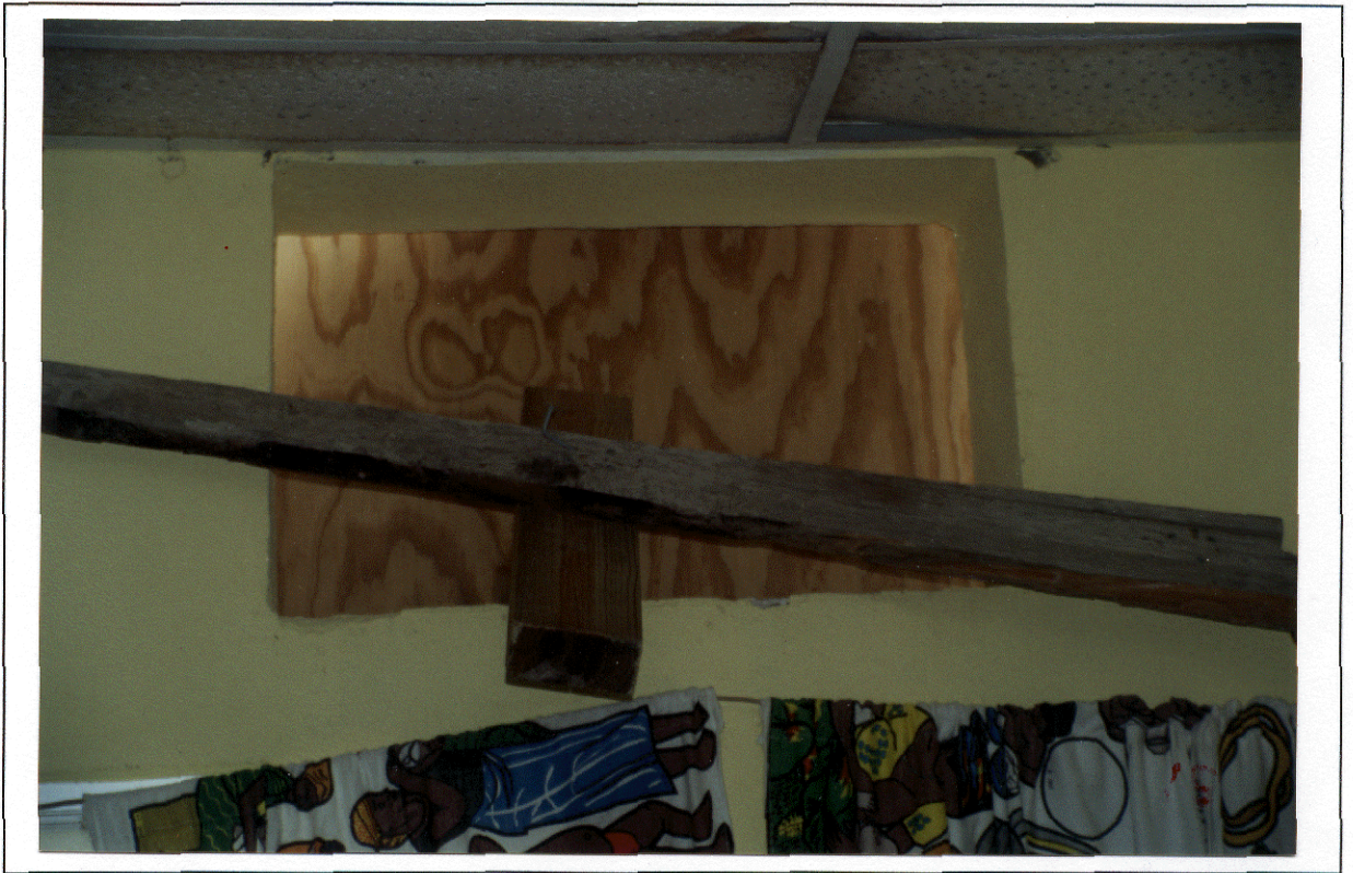
Photo 19 - Staff room Temporary closure of aperture for missing airconditioning unit
