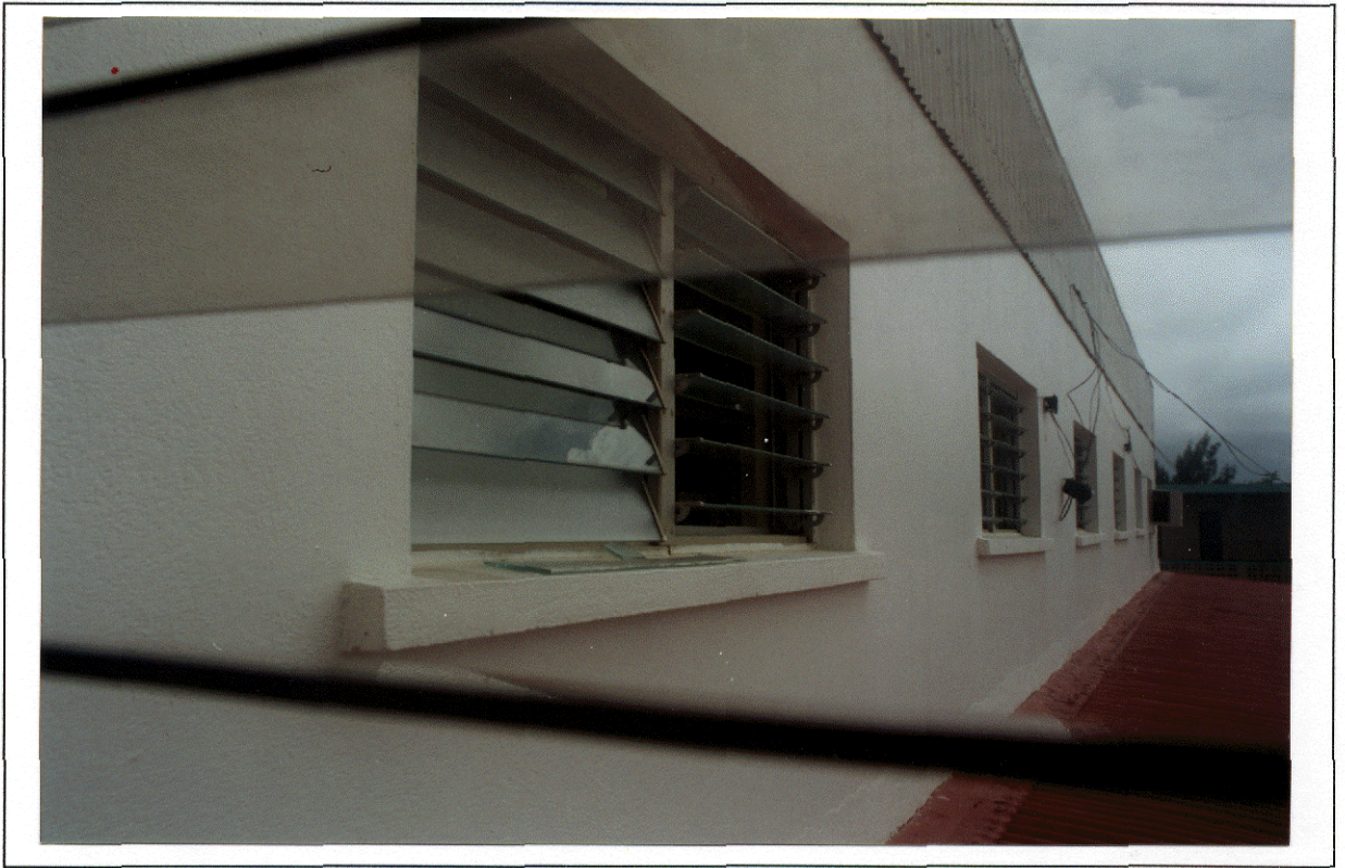
Photo 21 - Glass louvres These provide inadequate protection against wind-driven rain and flying debris.
