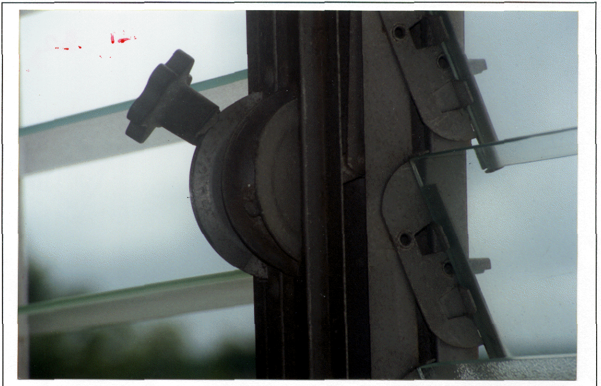
Photo 22 - Louvre-window hardware Several devices were broken thus rendering the closing of louvres difficult.
