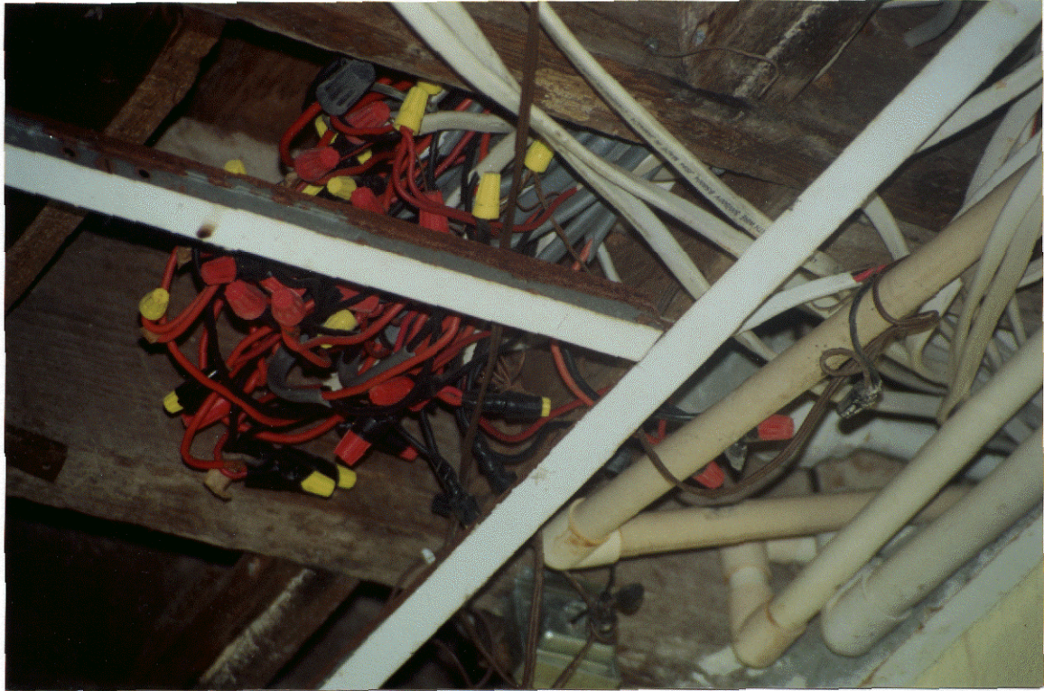
Photo 30 - Services Power, telecommunications and water in close proximity
