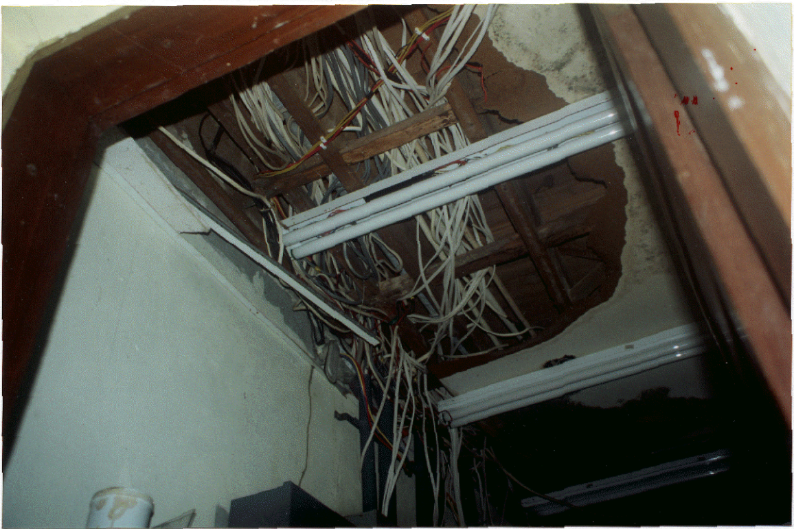
Photo 29 - Pump room Electrical wiring – Untidy, chaotic, unsafe?
