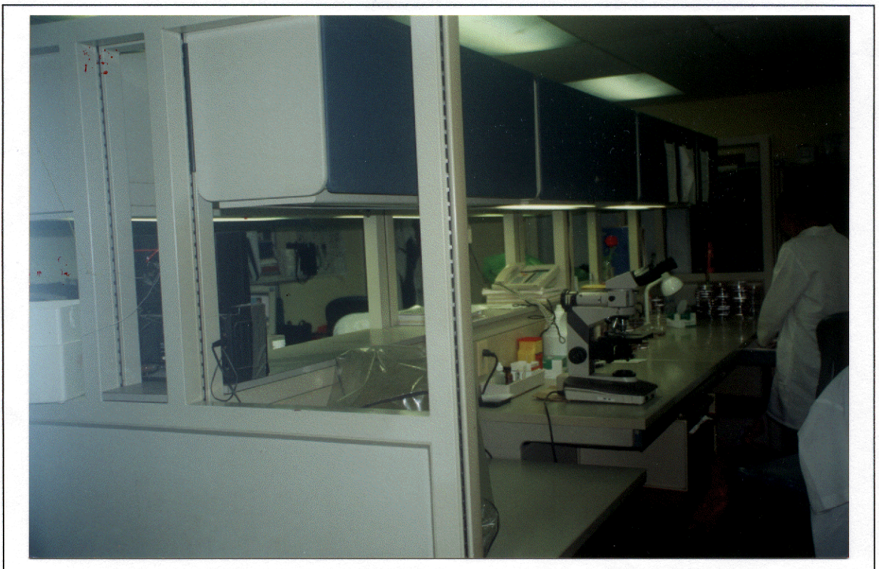
Photo 32 - Microbiology High-level cupboards kept closed to protect contents in the event of an earthquake.
