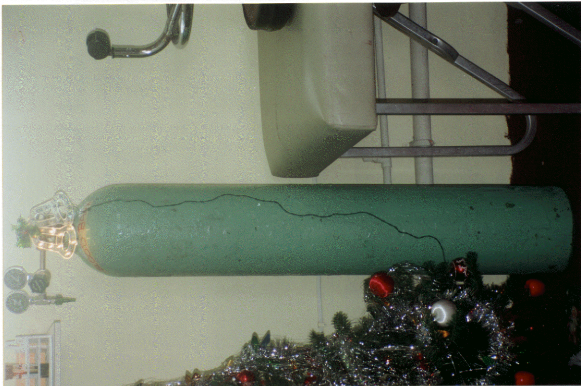
Photo 33 - Blood Bank Unrestrained gas cylinder is vulnerable to toppling in the event of an earthquake.
