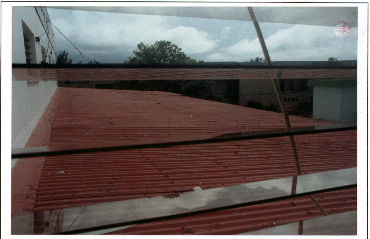
Photo 4 - The lower roof Arc-tangent, steel sheets cover original concrete roof
