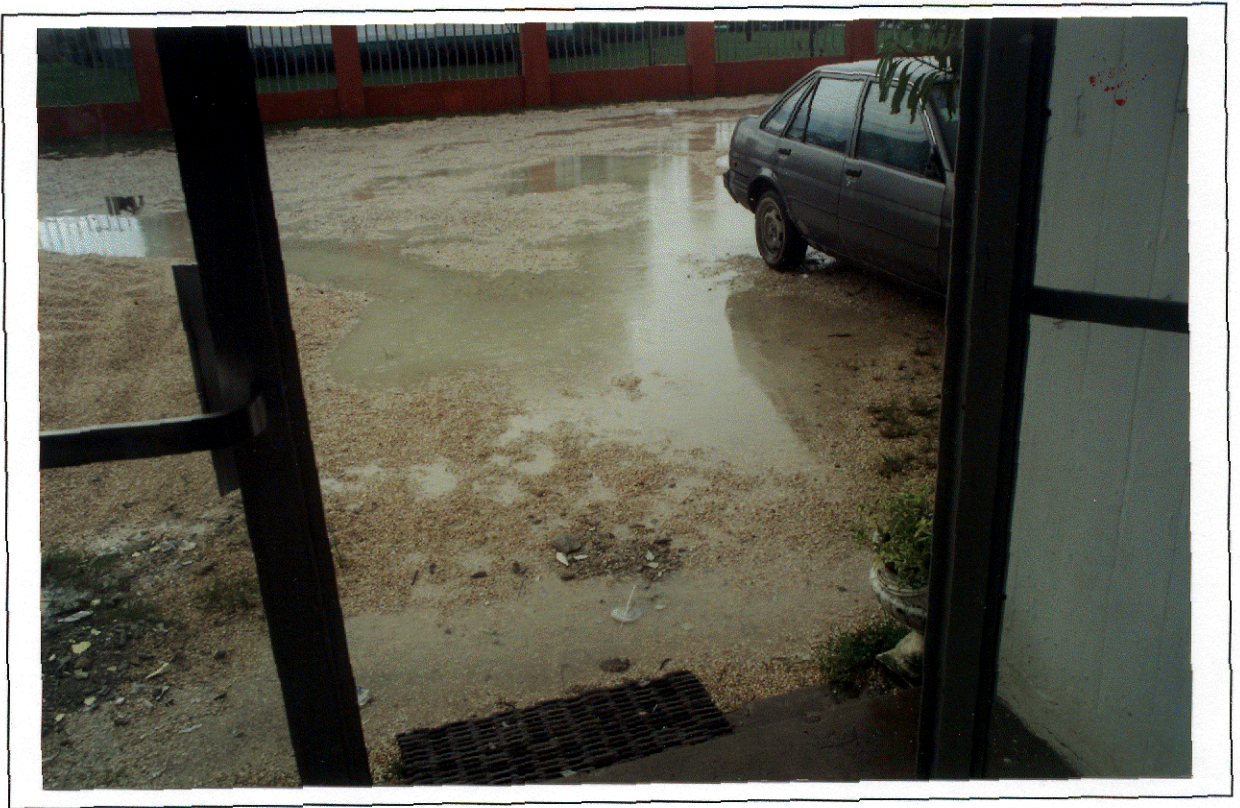
Photo 7 - Main entrance Low-lying and poorly drained
