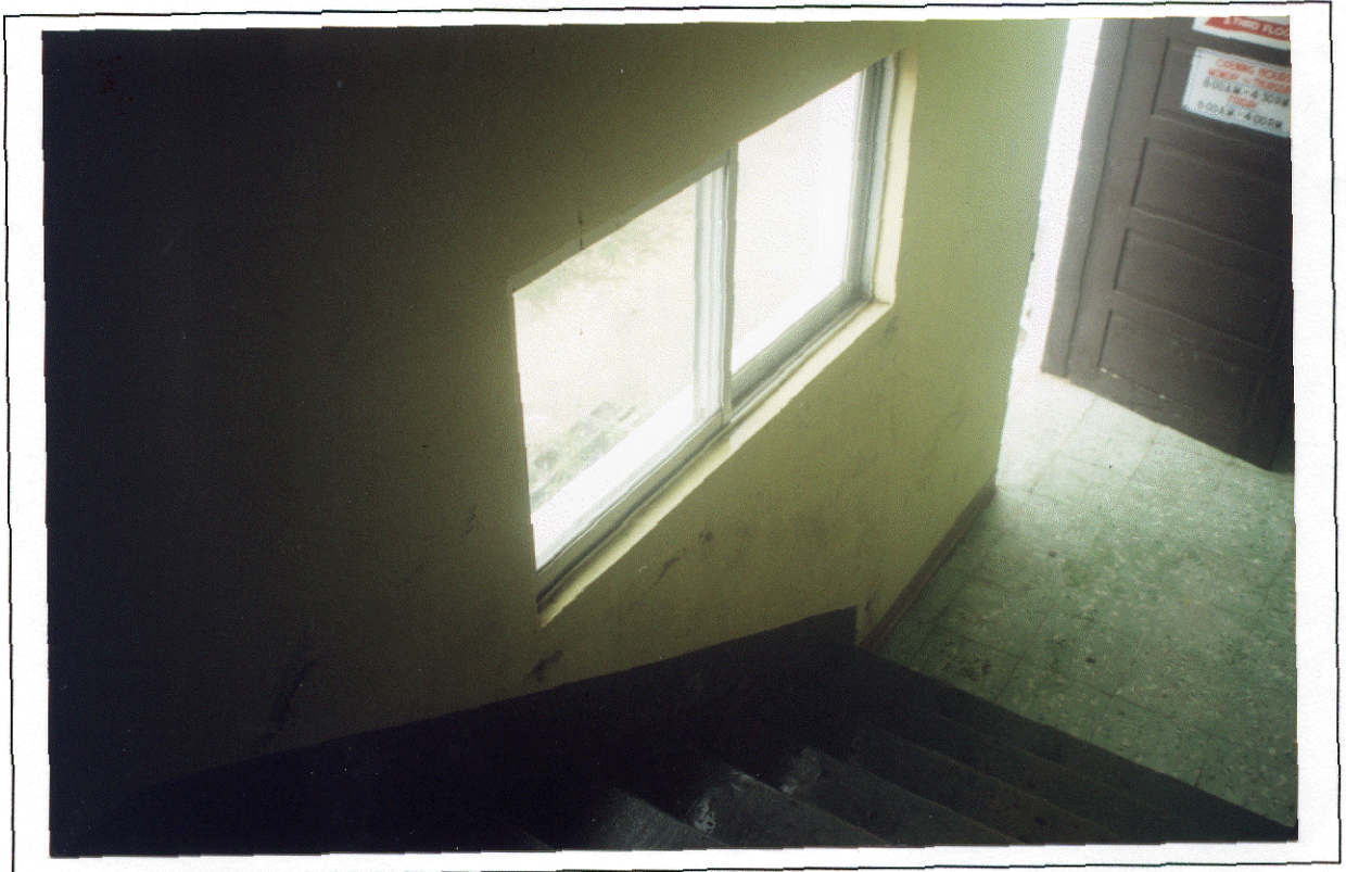
Photo 8 - Side entrance Wind-driven rain leaks through the windows
