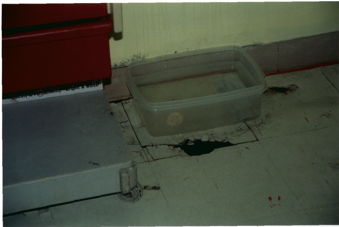
Photo 12 - Cytology Lab Basin collecting rain water because of leaks
