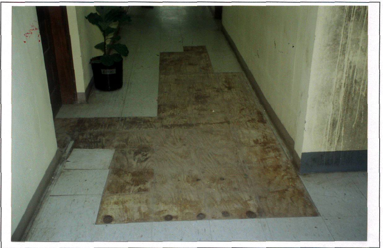
Photo 13 - Corridor Leaks led to loosening and removal of floor tiles
