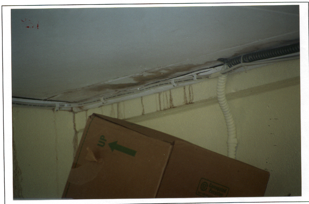
Photo 16 - Leaking at the perimeter
