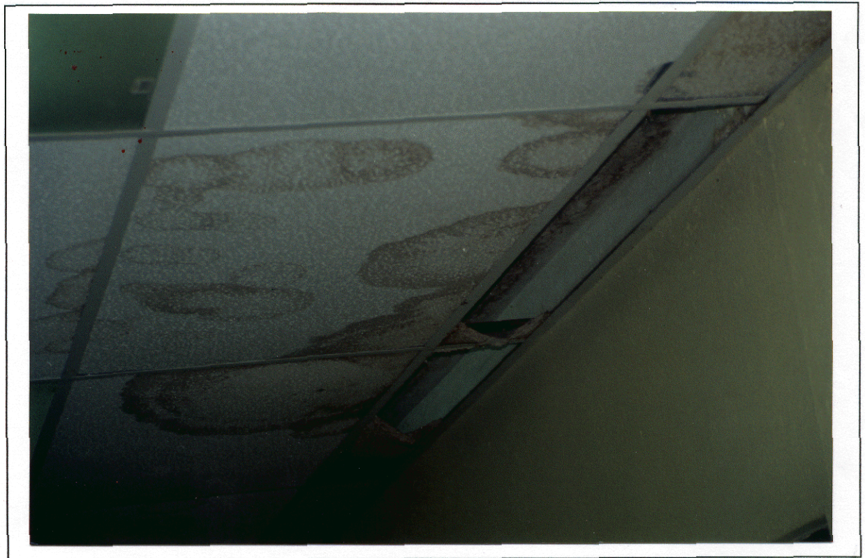
Photo 18 - Water-damaged ceiling There was extensive damage to ceilings and floor coverings.
