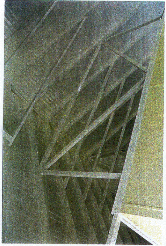
Photo 24: Typical roof truss in Private Ward.
