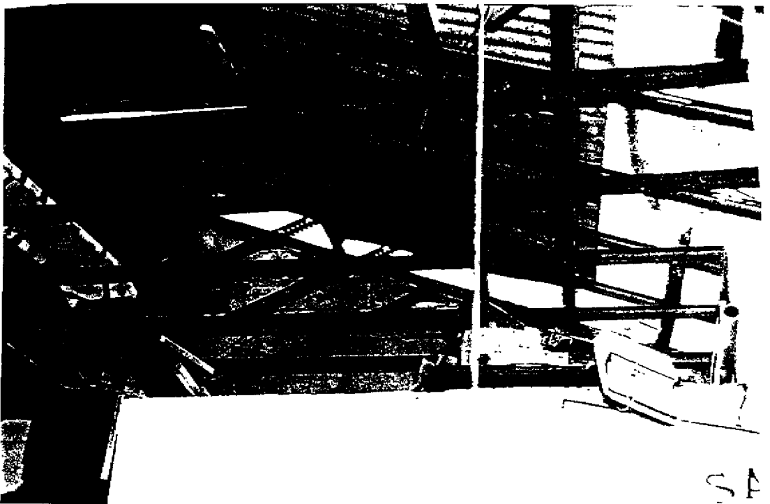
Photo HW-1. Rusting roof structure.
