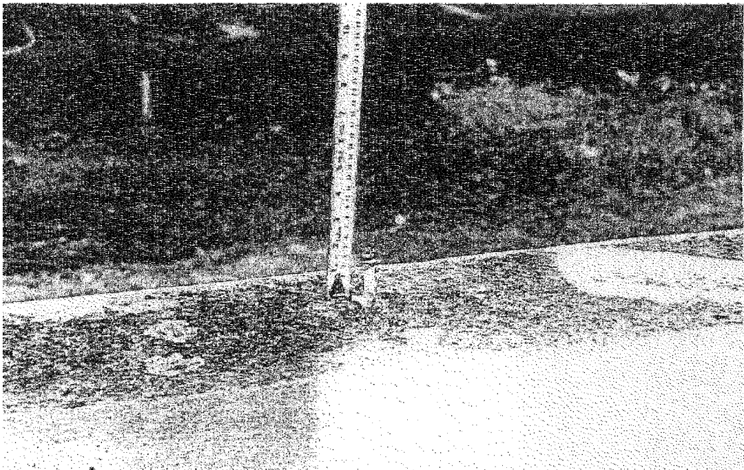
Photo HB-2: Wall plate stripped of wall, leaving the anchor bolt.
