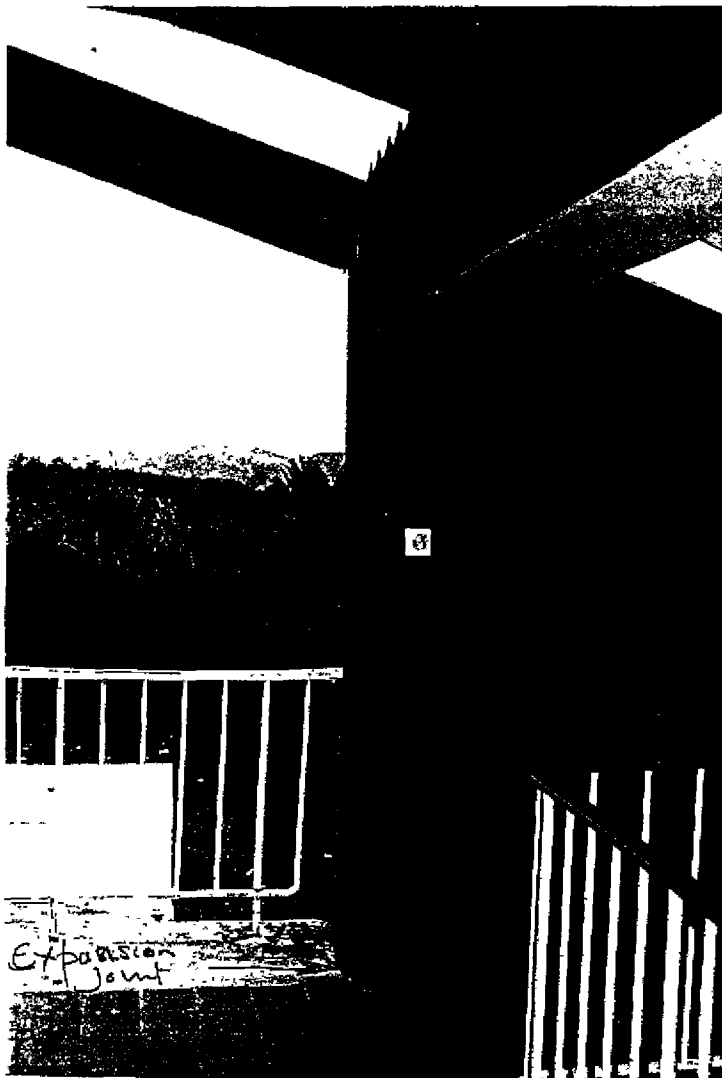
Photo HN-2: Expansion joint, no separation at roof level.
