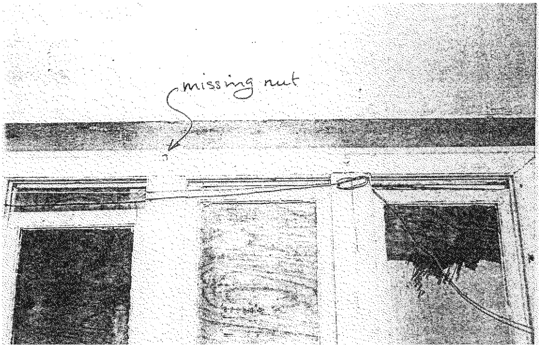
Photo S-3: Missing nut.
