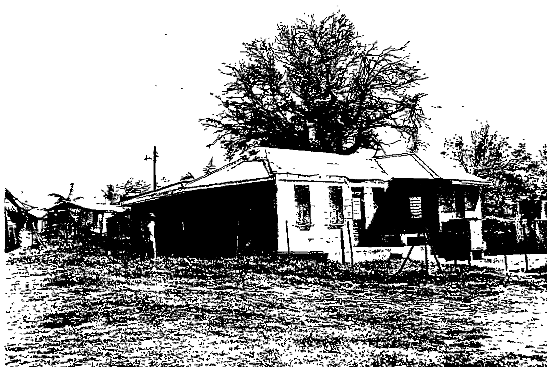
Photo C-1: Verandah roof and section of the main roof sheeting lost.
