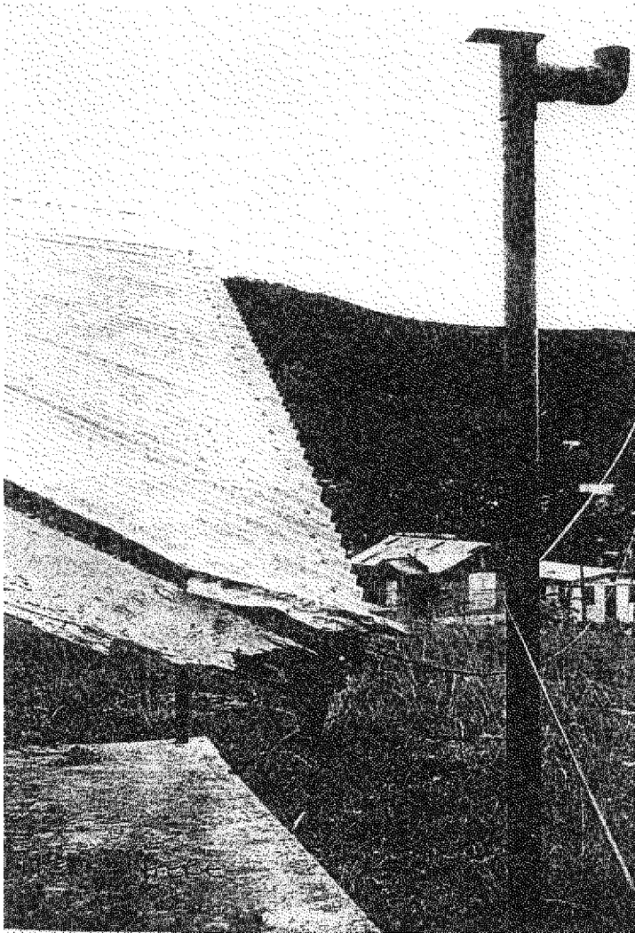
Photo JH-4: Rotten end of support to patio roof.
