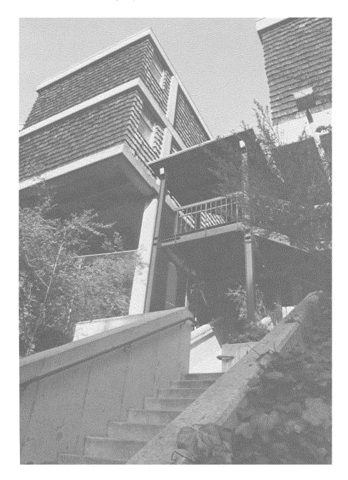
Berkeley's newest school, Cragmont, is a non-ductile concrete frame building. Features of its construction include cantilevered sections and a partial soft story.
