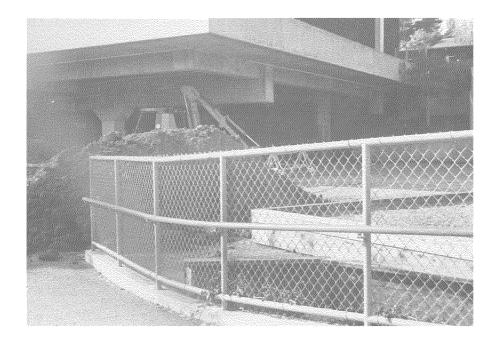
Because Cragmont is located very near the Hayward fault, it was important to trench on the property to determine the actual location of the fault.
