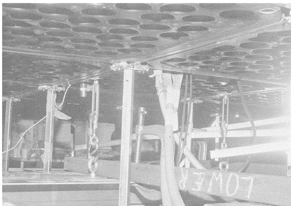
Fig. 3-6 Toggle Bar Installation
