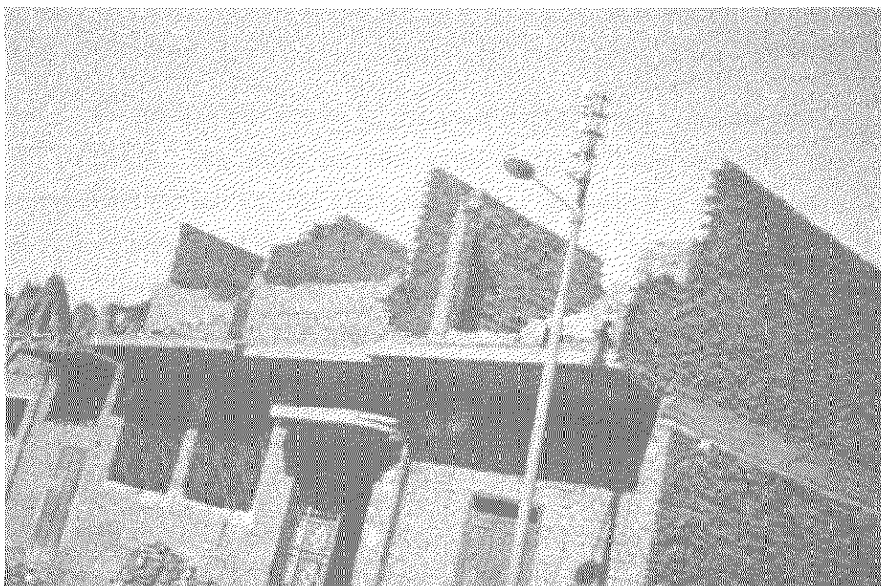
Figure 3-1a: Damage to unreinforced masonry buildings.
