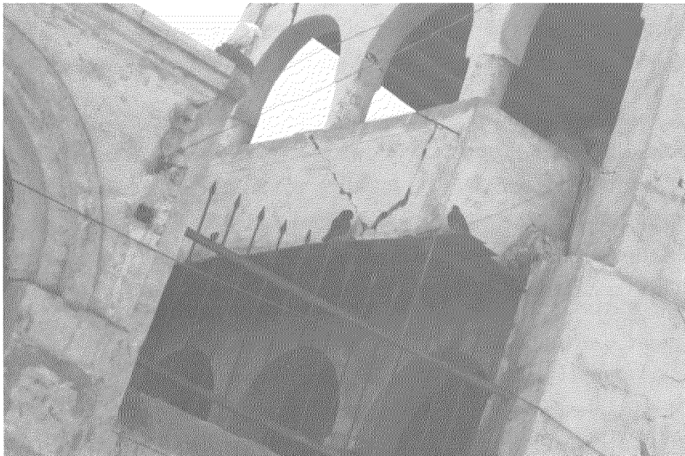
Figure 3-1b: Damage to unreinforced masonry buildings.
