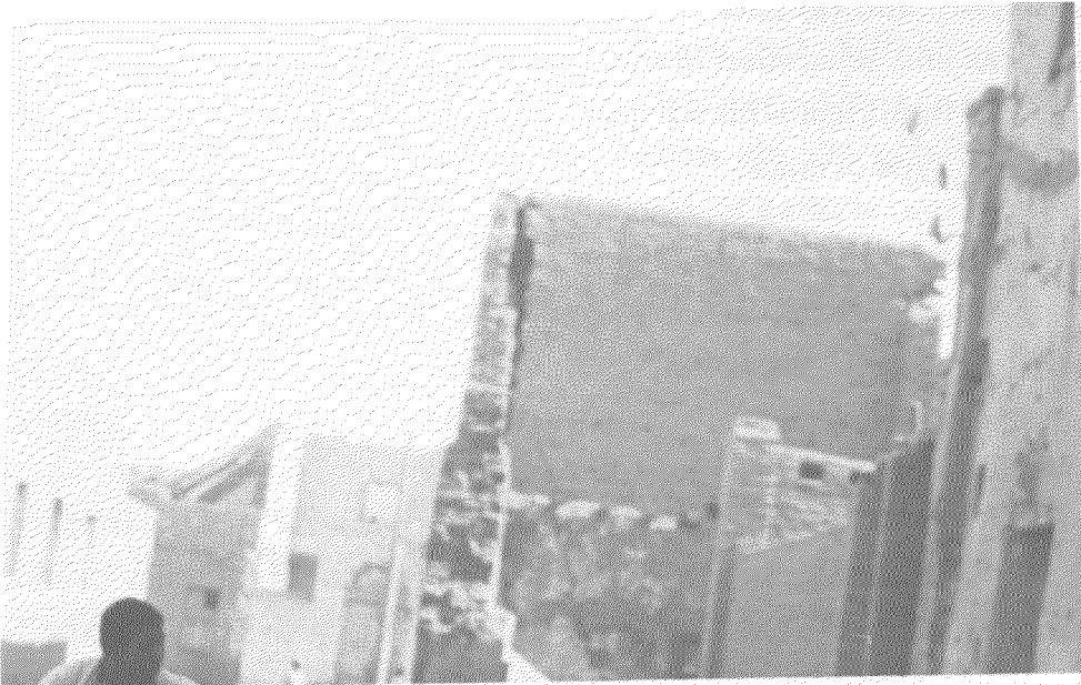
Damage to laterally unsupported walls and vertical cracks at wall connections due to lack of adequate anchorage.
