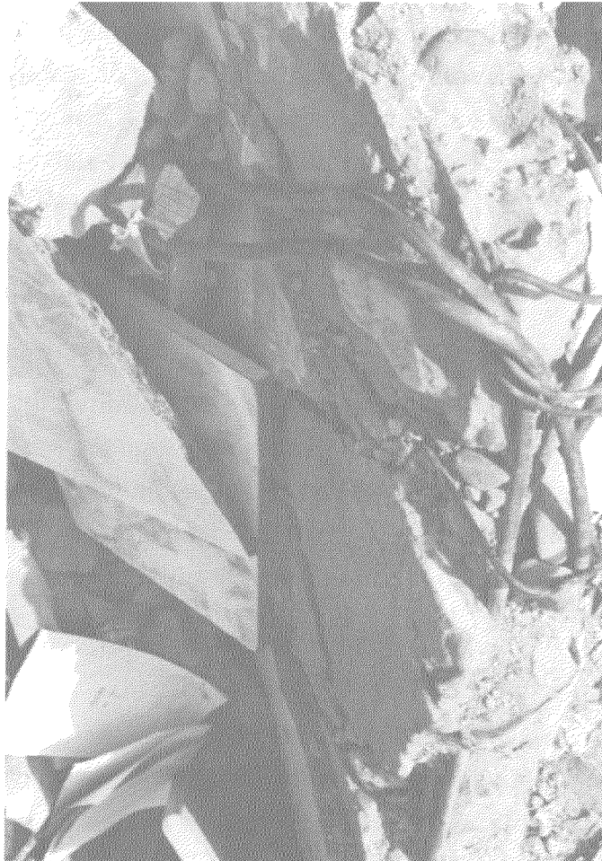
Figure 3-2: Collapse of a 14-story concrete-frame building.
