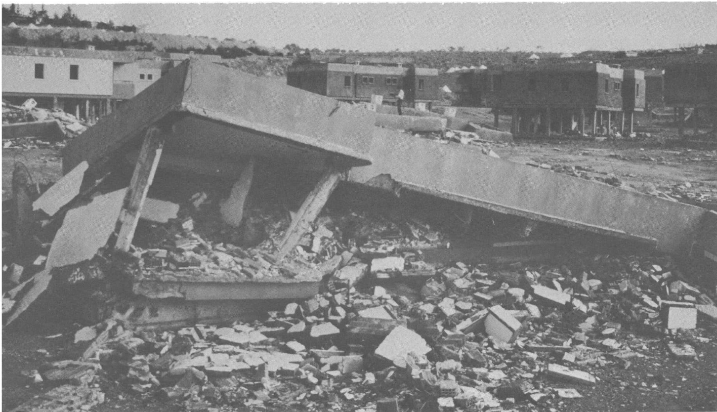
Fig. 2. Typical example of how buildings should not be built in earthquake zones. The picture shows some of the buildings in a large housing colony in El Asnam, Algeria, which were affected by the earthquake of about M 7.2 in October 1980. These buildings are top heavy and have a soft ground floor, the main reason for the extensive damage they suffered. This average damage amounted to 75 percent. Fortunately the buildings were still in the final phase of construction and had not yet been occupied.
