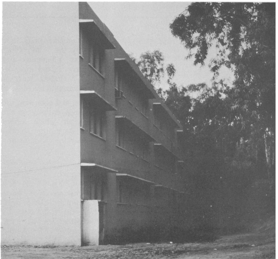
Fig. 3. This building not far from those shown in the previous illustration withstood the earthquake very well as did many others which were of a symmetrical and sturdy design without large openings.
