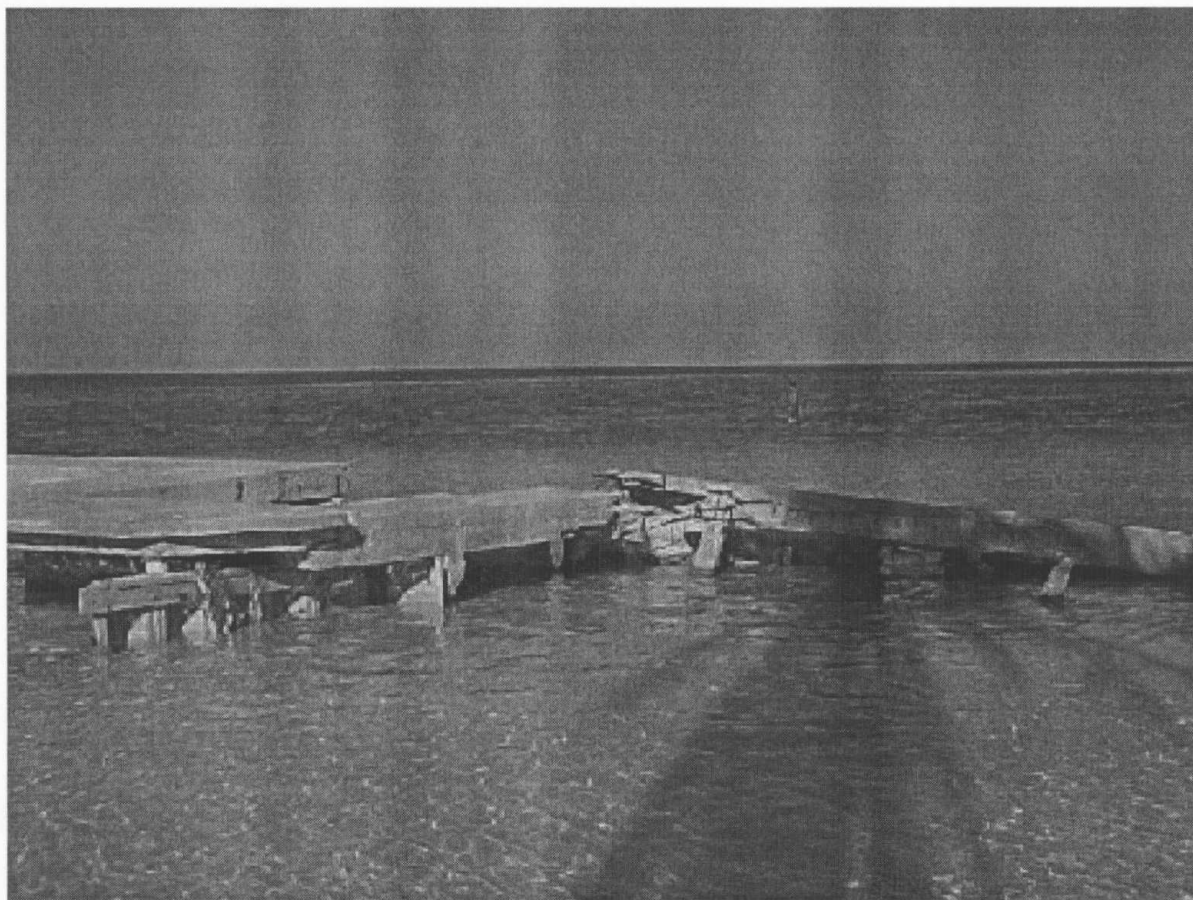
13. Caye Caulker: The split opened by Hurricane Hattie in the sixties grew wider, damaging existing seawall.
