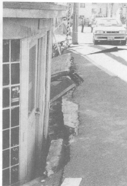
Photo 2 Settlement of building 8) (B in Figure 4)
