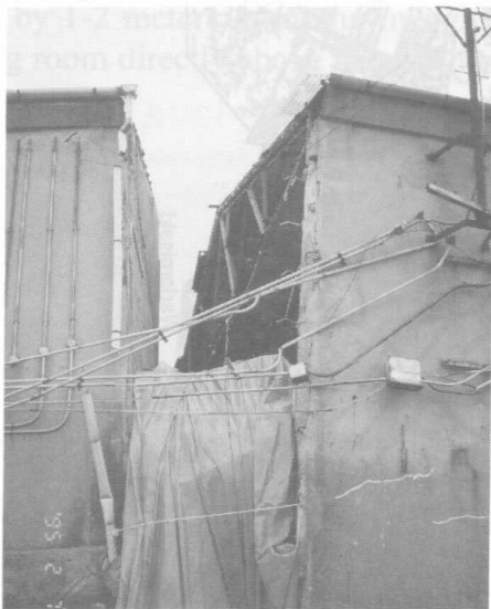
Photo 5 Separation of warehouse due to horizontal ground displacement (C in Figure 4)
