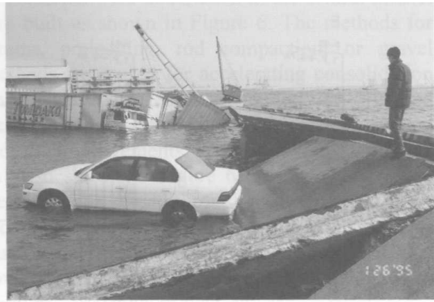
Photo 8 Submerged Pier No.5 of Kobe Wharf (F in Fig. 4)
