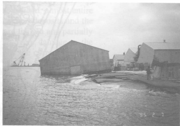
Photo 4 Submerged quaywall (C in Figure 4)
