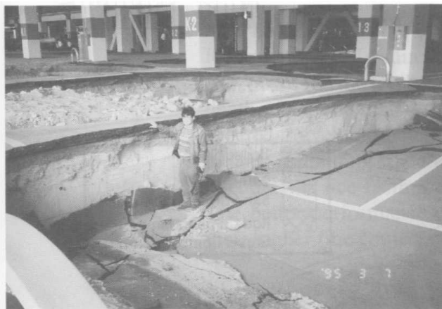
Photo 9 Settlement of parking area (G in Figure 4)
