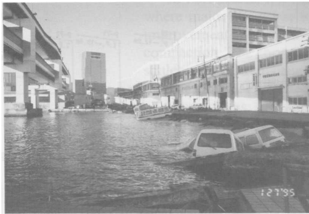
Photo 7 Submerged quaywall northeast of American Park (E in Figure 4)
