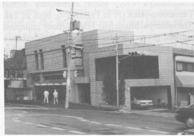
Photo 29 Liquefaction-induced settlement of stores near Torishima Dike (18)
