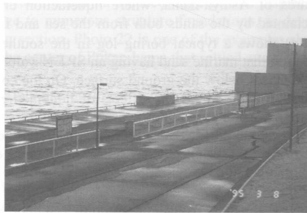
Photo 27 Quaywall of Naruo-hama where no major damage was observed ( W in Figure 4)
