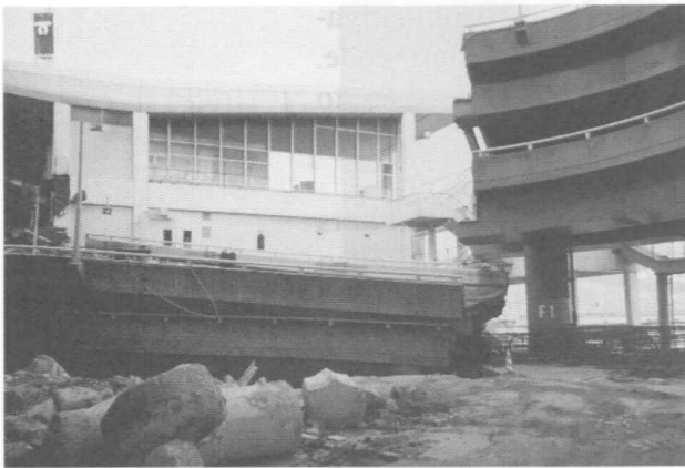
Photo 32 Bridge girder dropped due to ground displacement (A in Figure 13)
