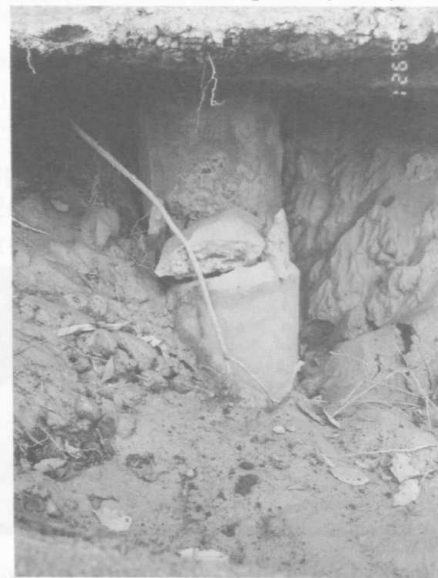
Photo 54 Concrete pile breakage due to ground movement (A in Figure 23)
