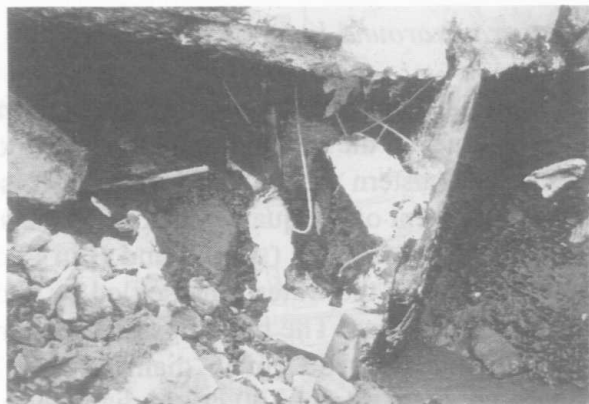
Photo 49 Failure of pile head due to lateral ground movement
