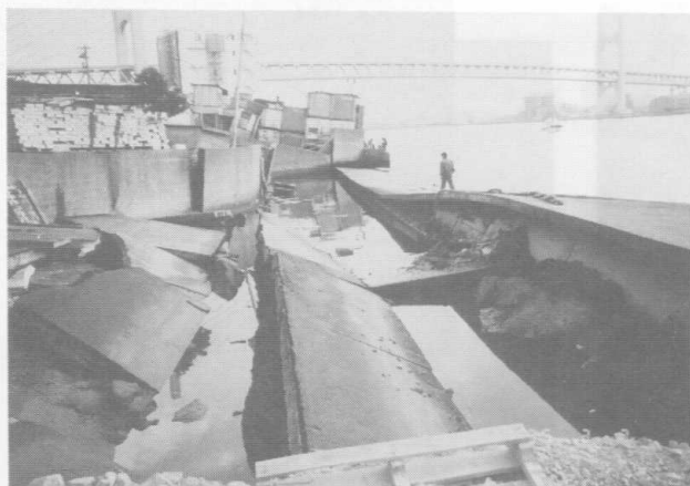
Photo 55 Large deformation of quaywall and ground behind the wall (A in Figure 24)
