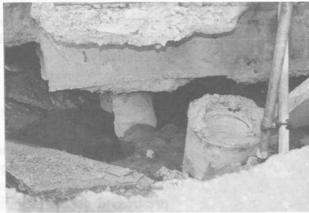
Photo 52 Separation of pile head due to ground movement (C in Figure 20)
