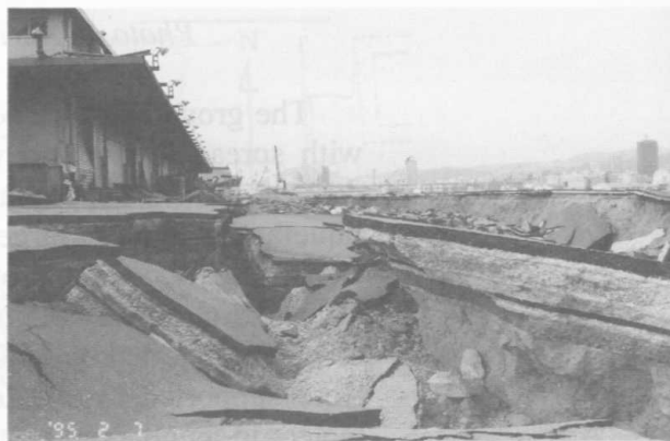
Photo 50 Large cracks and settlement of the ground behind quaywall due to lateral movement of the ground toward the sea (right)
