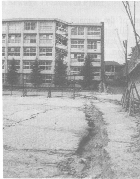
Photo 58 Collapsed school building due to lateral ground movement
