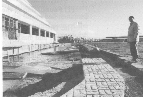
Photo 61 Ground in front of the hotel moved towards the sea and subsided
