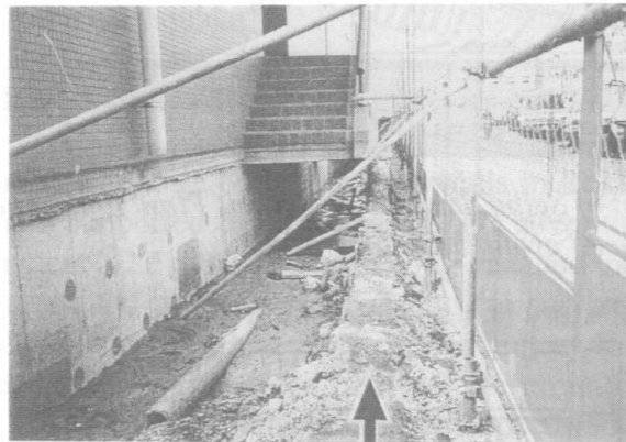
Photo 59 Inground wall of Shimagami Pumping Station, which appeared after the earthquake due to ground subsidence
