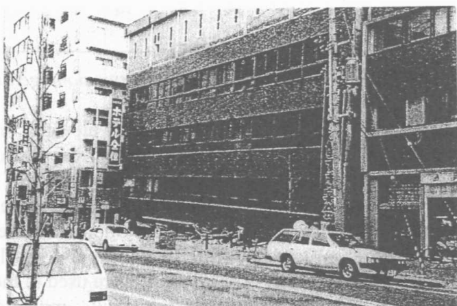
Photo 2 Damage to the first floor collapse-type
