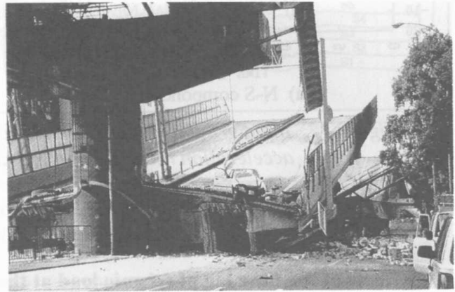
Photo 4 Damage to elevated expressway bridges (Fallen two adjacent simple-beam decks)
