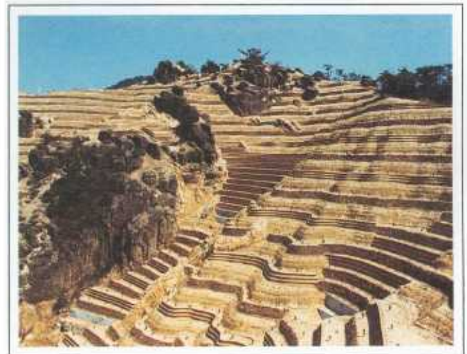
FIGURE 4.3 Afforestation by terracing. Location: Shiga, Japan Photo: M. Watanabe.
