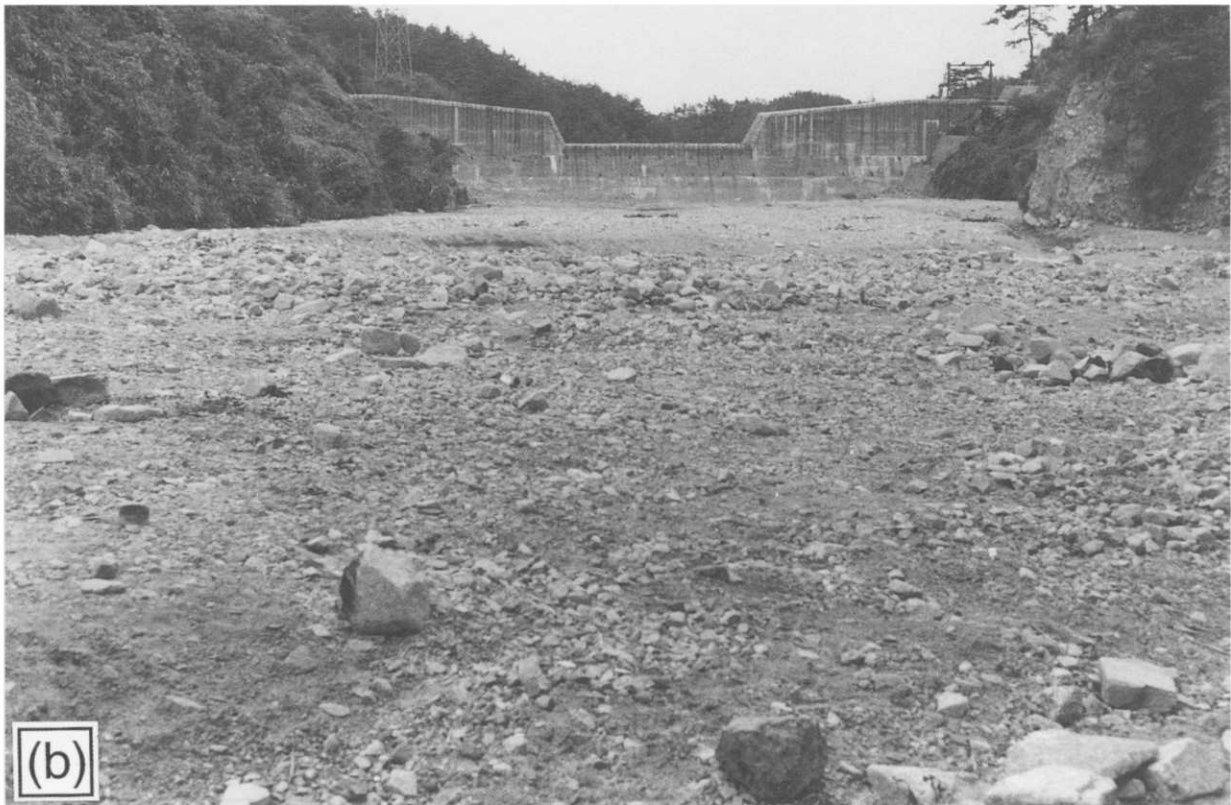
(b) After becoming filled with debris on 12 July 1967 Location Hyogo, Japan Photo, M Watanabe
