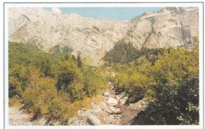
FIGURE 4.4 Ground sills to stabilize talus deposit. Location: Valais, Switzerland. Photo: M. Watanabe.
