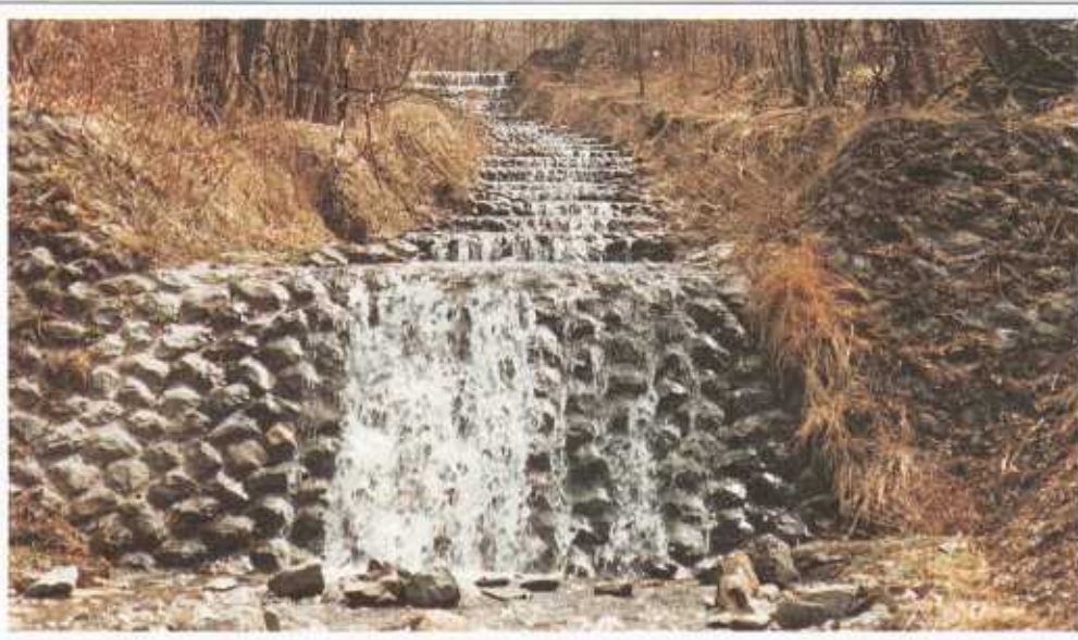
Figure 4.7 Check dams to stabilize the mobile material along a river valley.
