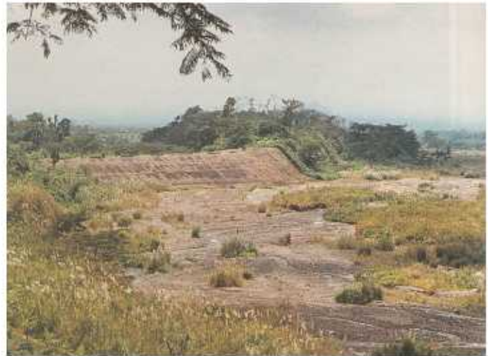
FIGURE 4.16 Diversion dam at Britar City. The dam blocks the channel towards Britar City. Location: East Java, Indonesia. Photo: M. Watanabe.
