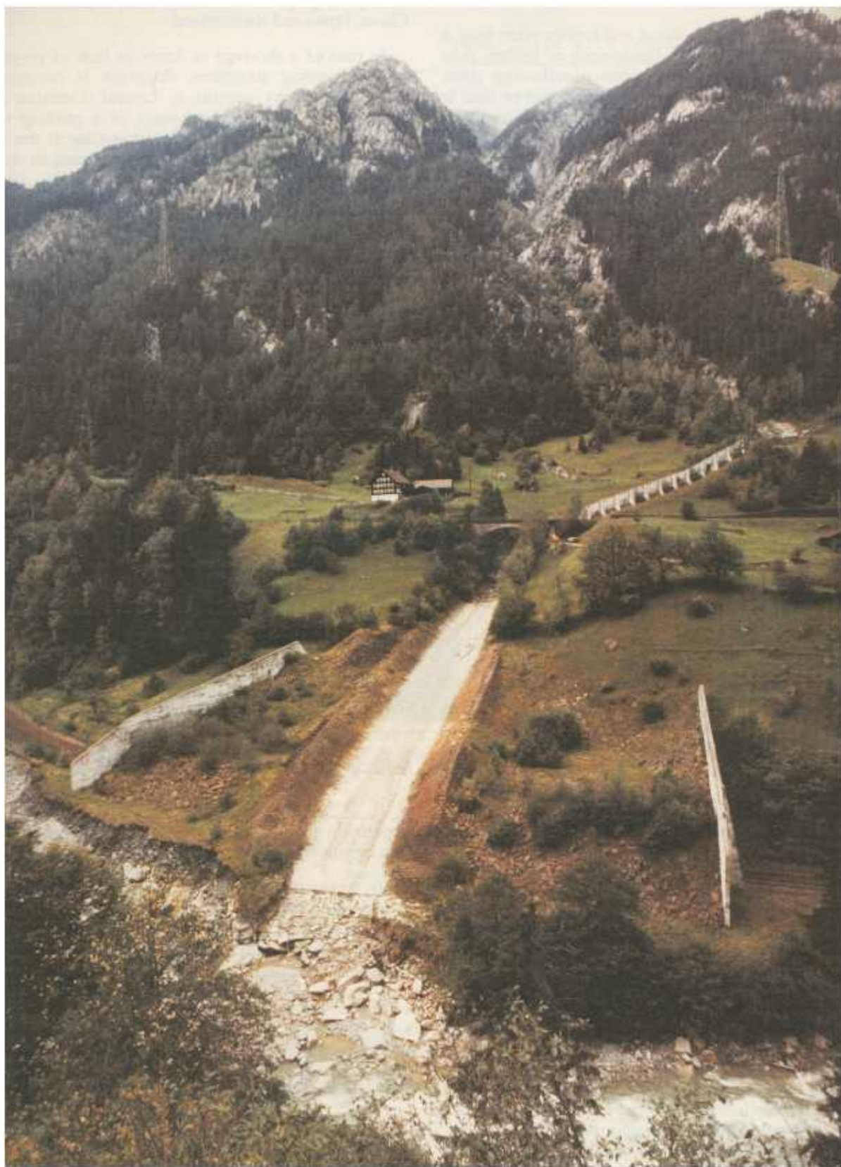
FIGURE 4.15 Flyover composed of guidewalls and a smooth channel. Location: Canton of Bern, Switzerland. Photo: M. Watanabe.
