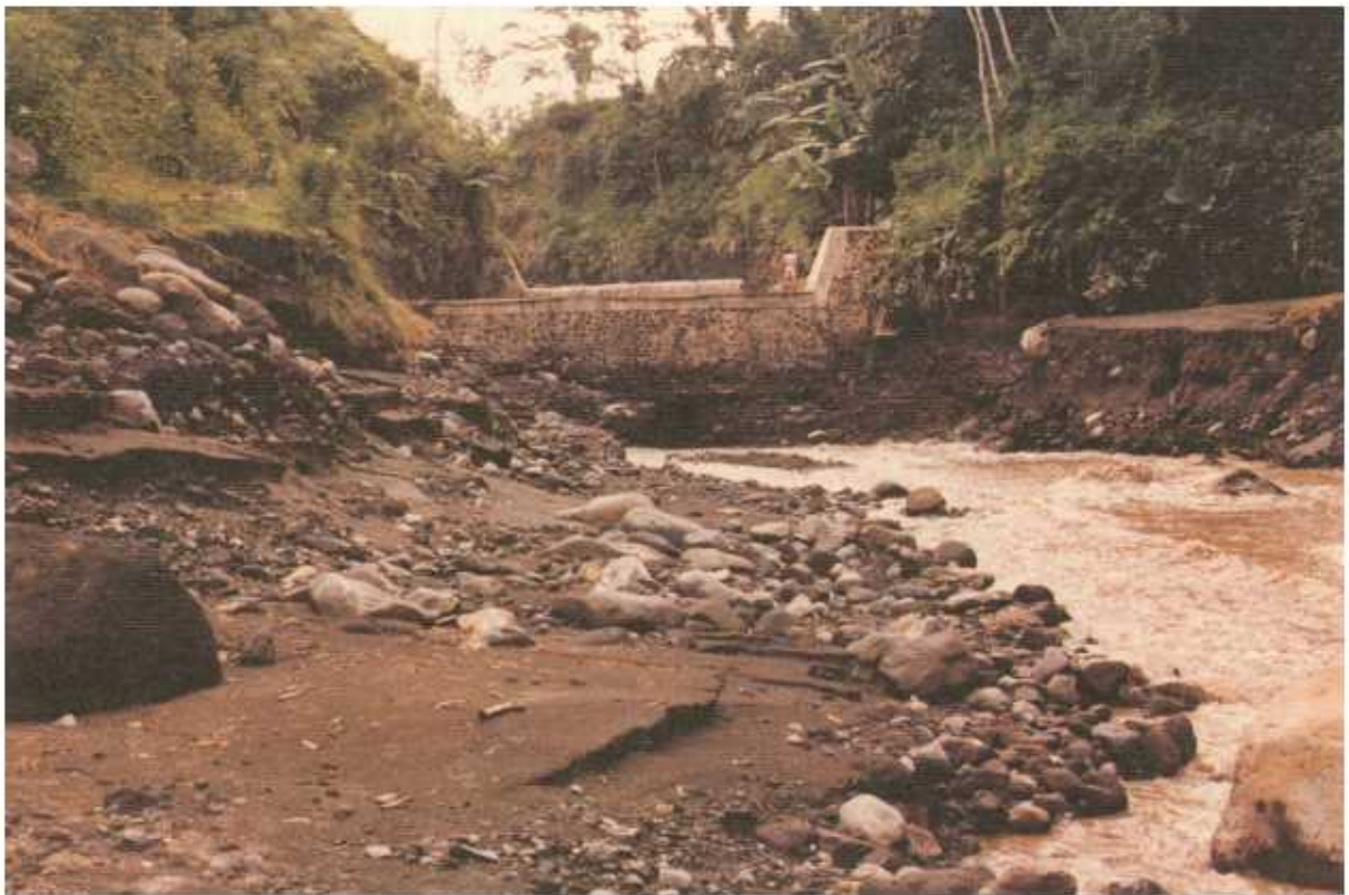
FIGURE 4.24 Check dam in which the foundation as a result of scouring disintegrated completely. Location: Yogyakarta, Indonesia. Photo: M. Watanabe.
