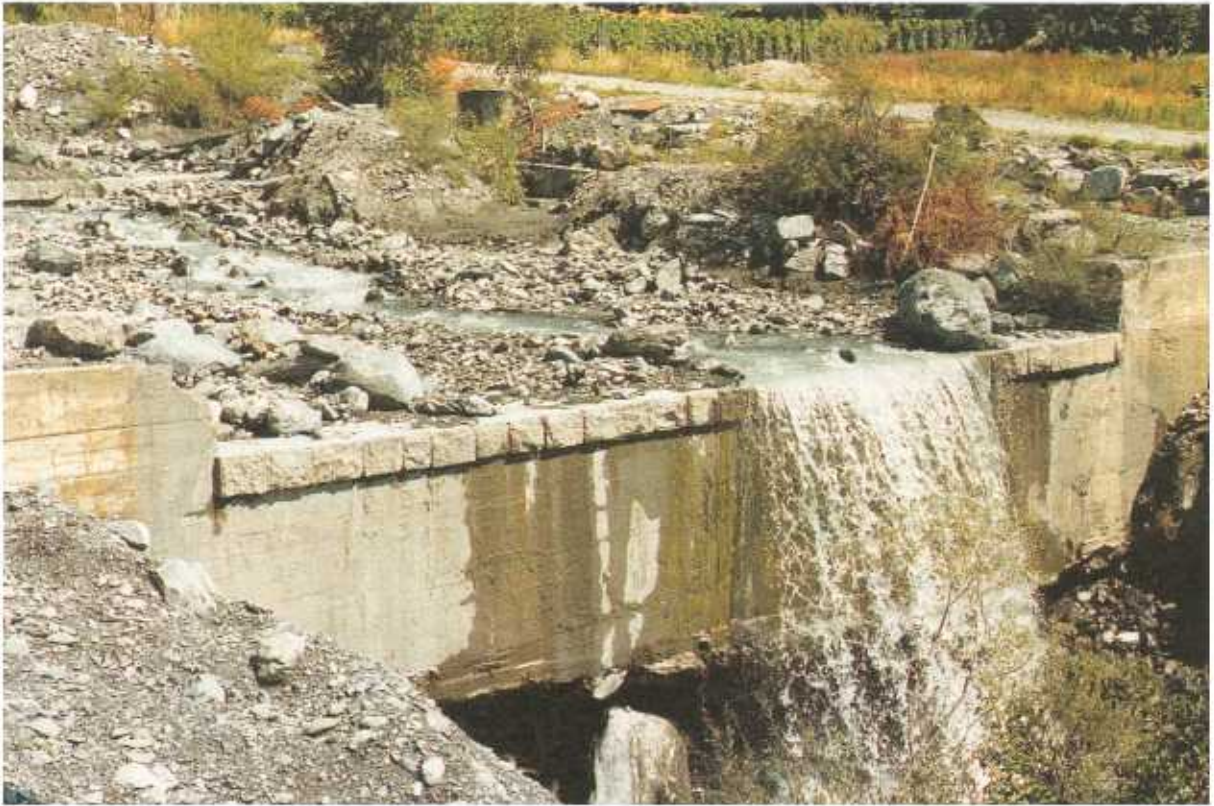
FIGURE 4.23 Poor design and construction always result in reduced efficiency and endanger the structure. Photograph shows ground sill endangered as a result of degradation and scouring. Location: Valais, Switzerland. Photo: M. Watanabe.
