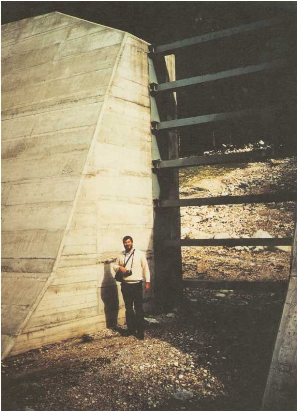
FIGURE 4.13 Screen attached to a check dam. Location: Canton of Zurich, Switzerland, Photo: F. Zollinger.
