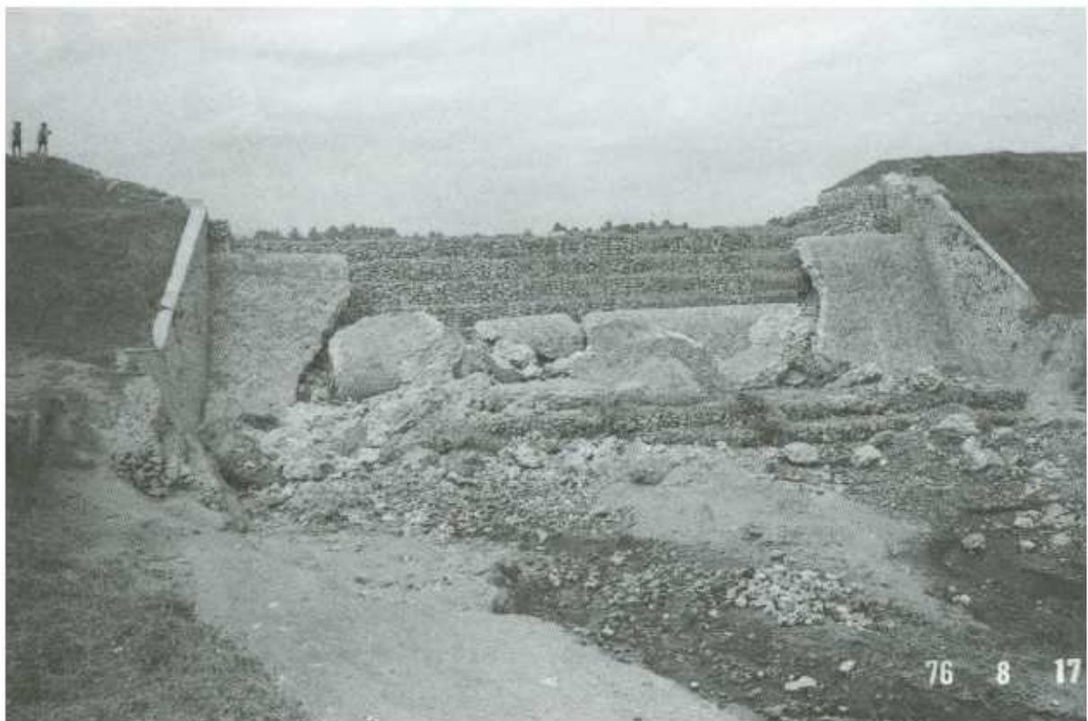
FIGURE 4.25 Outlet of a sand pocket where the toe of the retaining structure was scoured. It is essential to construct a pool at the toe of the dam in order to avoid local scouring caused by flood water. Location: East Java, Indonesia. Photo: M. Watanabe.
