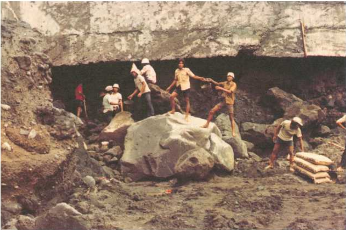
FIGURE 4.26 Destruction caused by scouring of the foundation of a check dam. Scour protection can be achieved by constructing a ground sill immediately downstream of the dam. Location: Yogyakarta Java, Indonesia. Photo: M. Watanabe.
