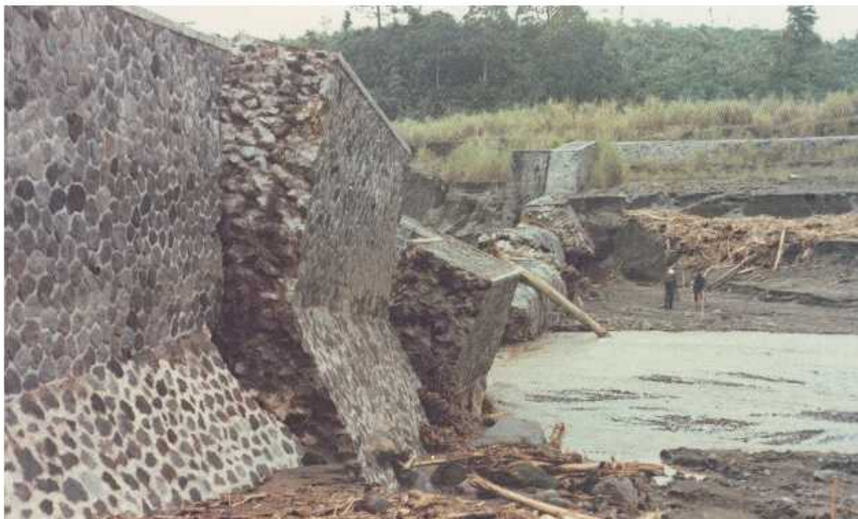
FIGURE 4.27 Check dam destroyed because of an inadequate foundation. Emergency filling work was required. Location, Central Java, Indonesia. Photo: M. Watanabe.
