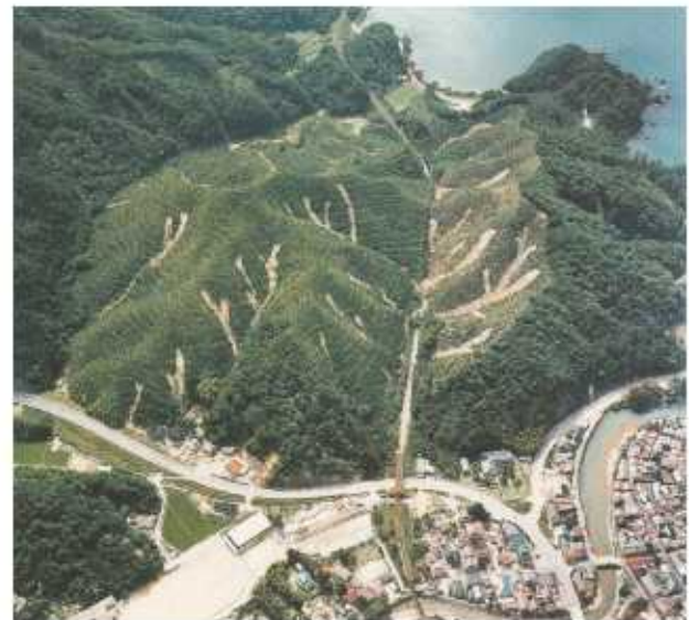
FIGURE 8.11 Remarkable contrast between clear-cut slopes and slopes with forest cover in terms of slope stability. Location: Nagasaki, Japan. Photo: M. Watanabe.
