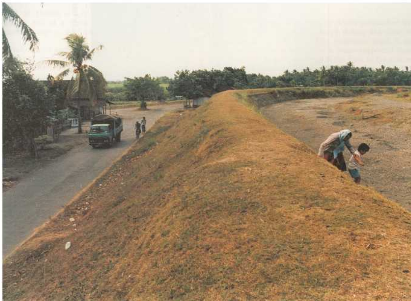
FIGURE 8.32 Brantas River. The bed level rose up to the ceiling level of a nearby house on the alluvial fan, after deposition by lahars from Mt. Kelut. Location: East Java, Indonesia. Photo: M. Watanabe.
